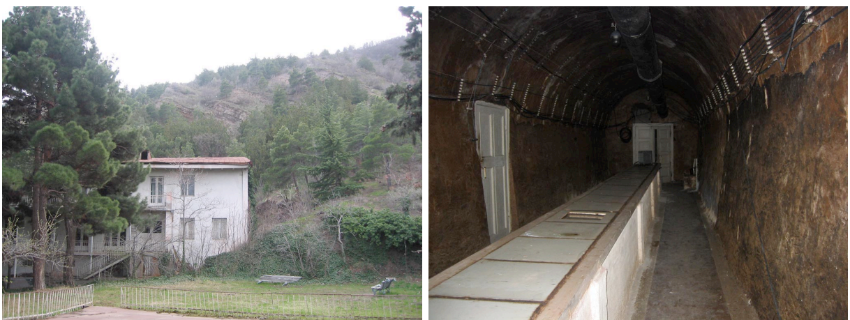
Fig. 7 Mtatsminda (TBL) Geophysical Observatory building and tunnel
